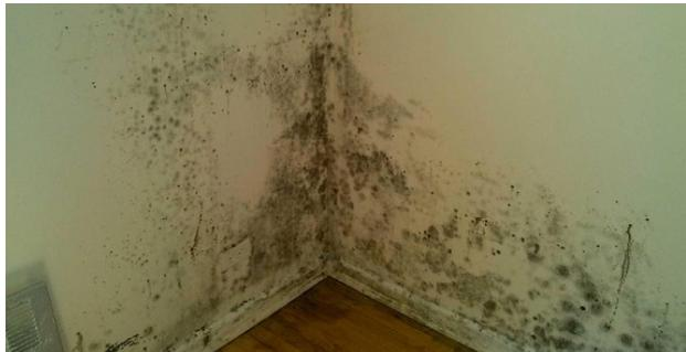
Given time, the affected damp areas then attract black mould that grows on the surface. Moisture from kitchens and bathrooms is a major cause and affects other colder parts of the property. Common causes include too much moisture being produced in your home, not enough ventilation and the temperature in your home not being kept on to an even level temperature. Condensation can be reduced by increasing ventilation and reducing the amount of moisture in the air.
